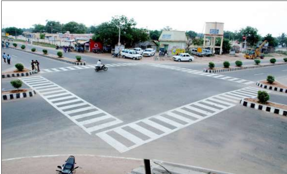
Improved Junction at km 25/8 of Pollachi – Dharapuram – Karur road
