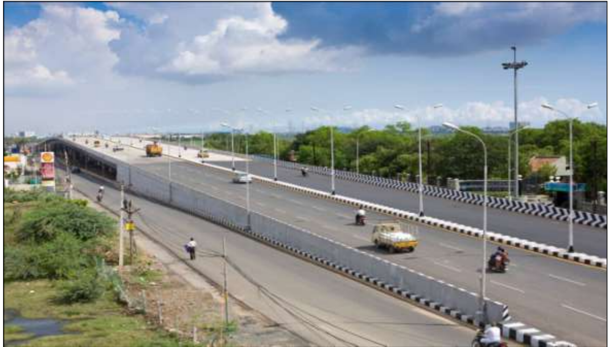
Road Over Bridge constructed at the junction of Velachery – Tambaram road and Pallavaram – Thuraipakkam road
