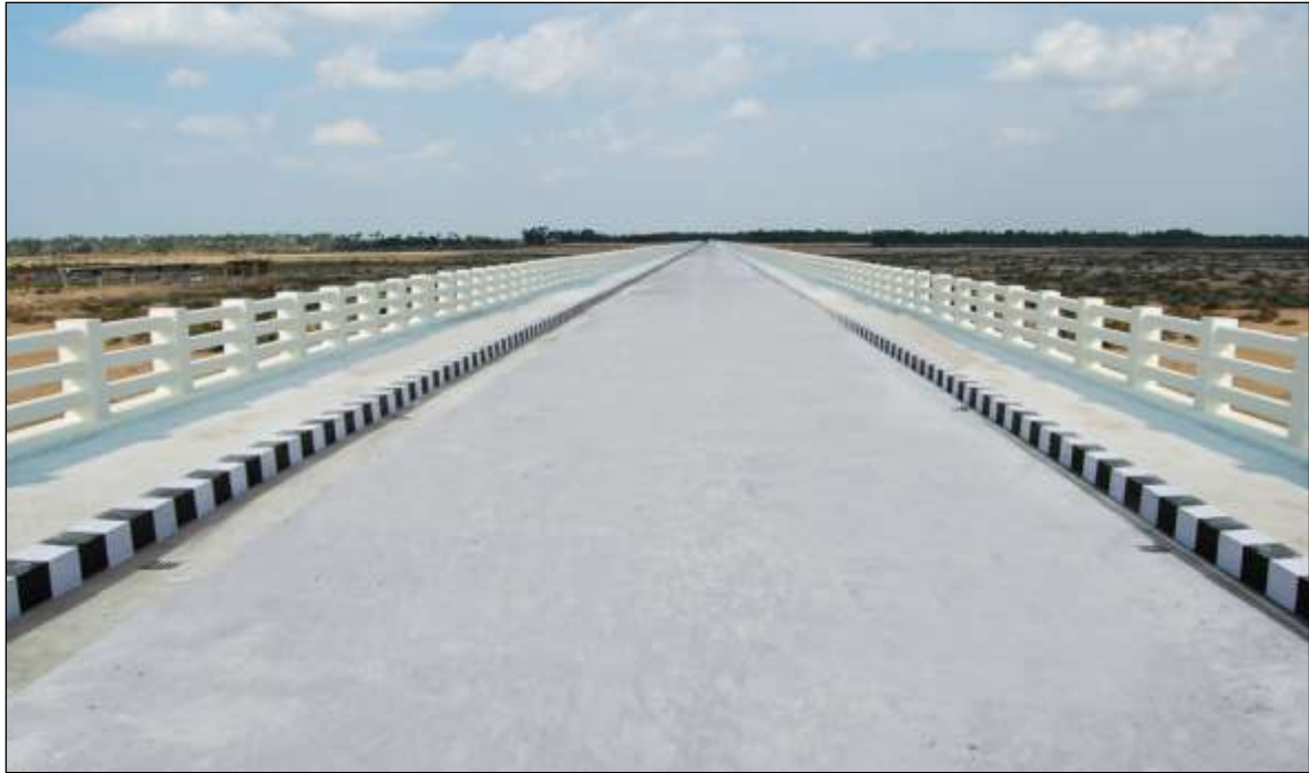
Bridge constructed across Kollidam river to connect villages Sengaraiyur in Trichy district and Alamelupuram Poondi in Thanjavur district
