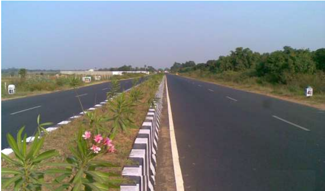
Garden maintenance in the centre median of Thirumazhisai – Sathiyavedu road
